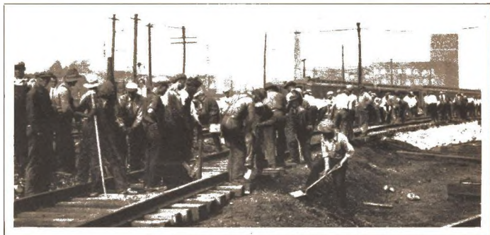
Laborers Re-lining Trackage Entering Montreal, as Part of the Construction Work of the Proposed New Canadian National Terminal
