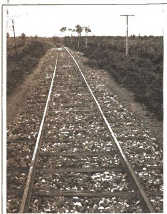
Ballast on the T. G. R., as Shown Above, Is Not Exactly the Kind That a Chesapeake & Ohio Section Boss Would Be Proud of
